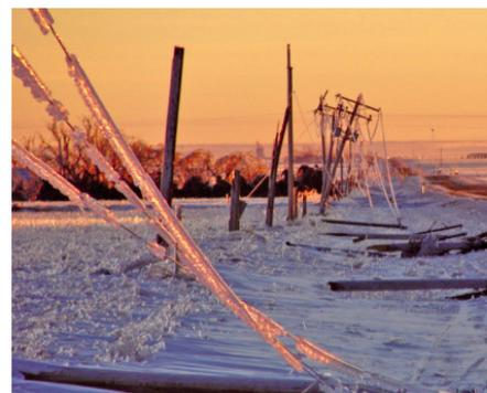
Non-VR2® cables fall to the weight of ice and force of wind. Photo taken by Ross Riley
