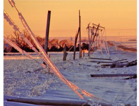
Non-VR2® cables fall to the weight of ice and force of wind. Photo taken by Ross Riley
