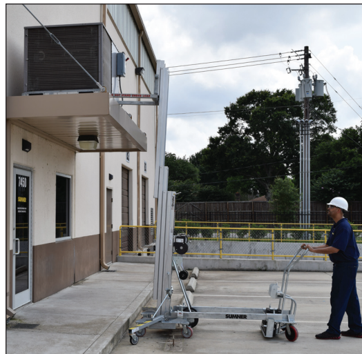
Works around ground obstructions
