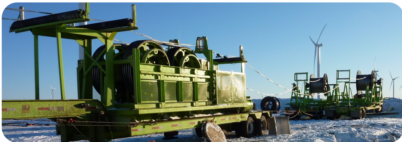
Figure 6: Payoff and bullwheel setup.
