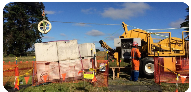
Figure 10: Suitable technique for roller diversion, courtesy of Transpower New Zealand.
