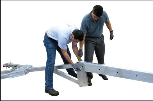
2. Lift one side of cross beam onto A-frame and line up outside bolt hole on A-frame with desired bolt hole on cross beam. Place bolt through bolt hole on A-frame and cross beam with washers on either side of the bolt. Loosely tighten so A-frame can swivel when A-frame is erected.
