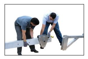
Place trolley at the opposite end of the cross beam. Center trolley on cross beam and tighten with set screw.
