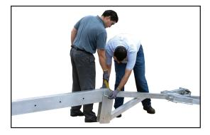
4. Lift cross beam end without bolt inserted and position on A-frame lining up outside bolt hole on A-frame with desired bolt hole on cross beam.
