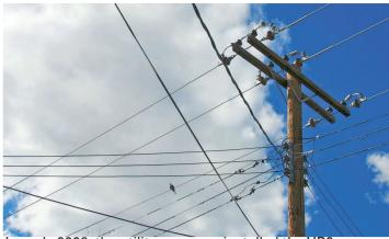
In early 2008, the utility company installed the VR2 conductors on a .65-mile stretch of 69 kV horizontal post insulator as a side-by-side comparison with traditionally-constructed twisted pair conductor on different phases of the three-phase line. VR2 cable is third from the left in the photo above. The traditional construction continued to exhibit bagging problems. The new VR2 went up without a hitch. "The difference was like night and day," says the project manager.
