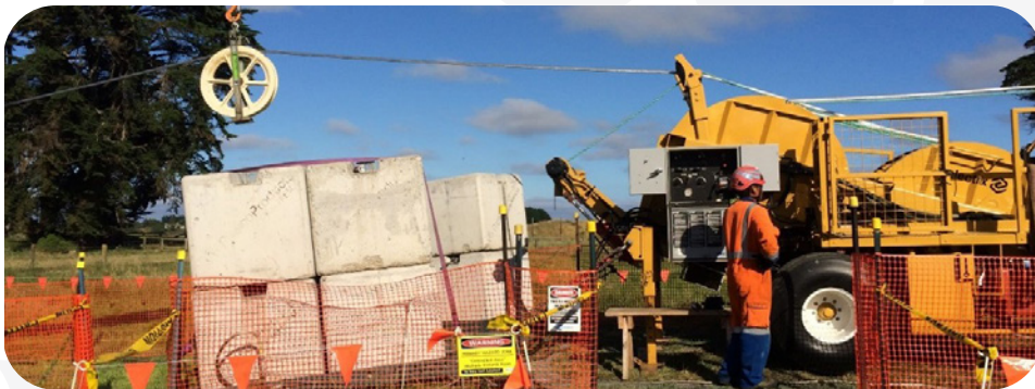
Figure 9: Suitable technique for roller diversion, courtesy of Transpower New Zealand.
