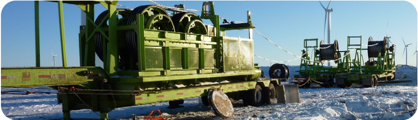
Figure 5: Payoff and bullwheel setup.
