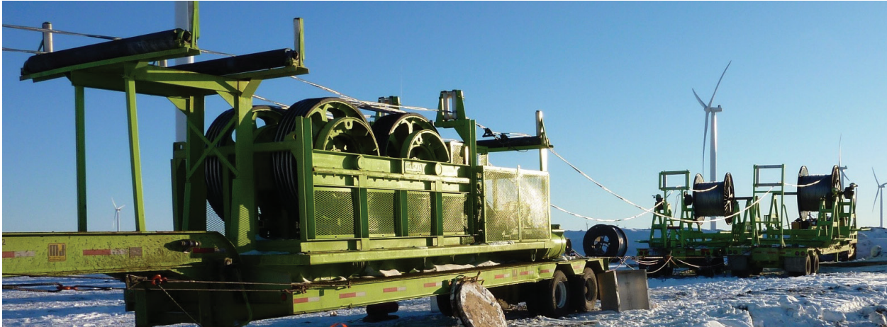
Figure 4. Payoff and bullwheel setup.
